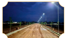
Complete Electrification & Street Lights
