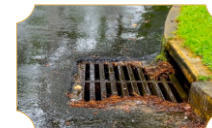
Storm Water Drainage System
